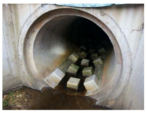
Figure 4-8: Baffle type fish passage installed at Waiwera
